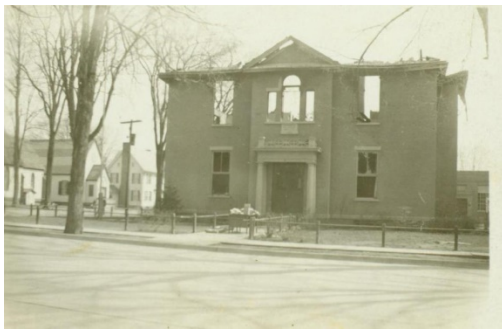
Fire at District 5 School
