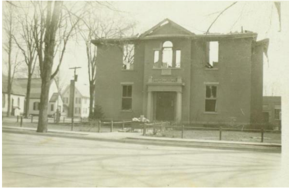
Fire at District 5 School
